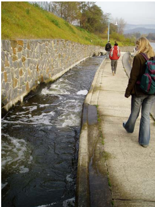
Fig 3 Fish-pass in Strekov dam, River Labe (2005)
