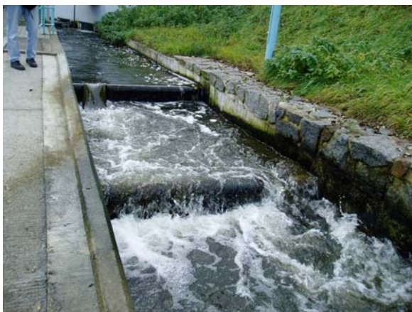
Fig 1 Chamber fish-pass in Strekov, Labe River (2005)
