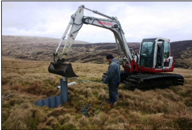
Piling to form a small dam, Whitendale, February '05
